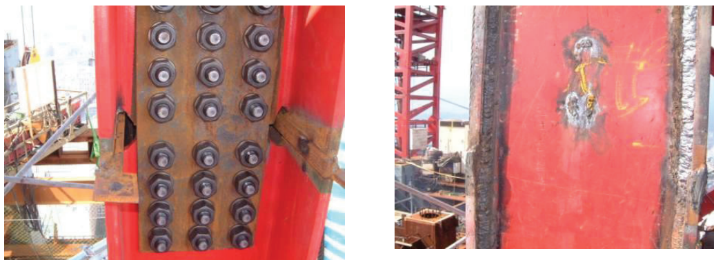
(a) Bolted web and welded flange
